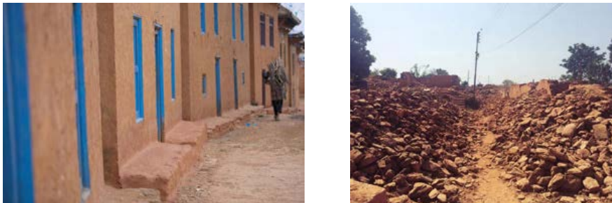
The charming village of Saathigar in Kavre district was reduced to rubble, as shown in this mobile-phone shot of the village after the quake. (Left photo: Thomas L. Kelly, right photo: Claire Burkert)
