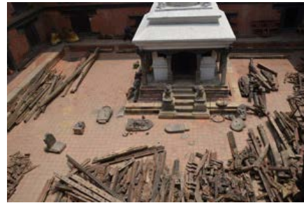
Left: A toppled temple pinnacle on the Patan Darbar, a World Heritage Site. Right: Struts, columns and stone sculptures from collapsed temples on the Patan Darbar were safeguarded in the Patan Museum. When the temples are rebuilt, consideration needs to be paid to strengthening them to withstand future earthquakes. (photos: Claire Burkert)
