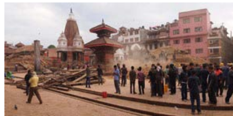
The two collapsed temples
