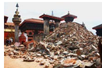
Bhaktapur Darbar Square with the collapsed sandstone temple of Vatsala Devi
