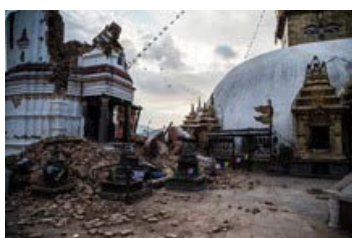
Severe damage of 17th century shrine of Anantapur at the Great Stupa of Swayambhu
